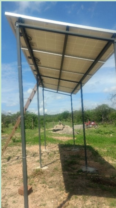
Image: Solar system for pumping (source: SOL Luções Energia Solar)
