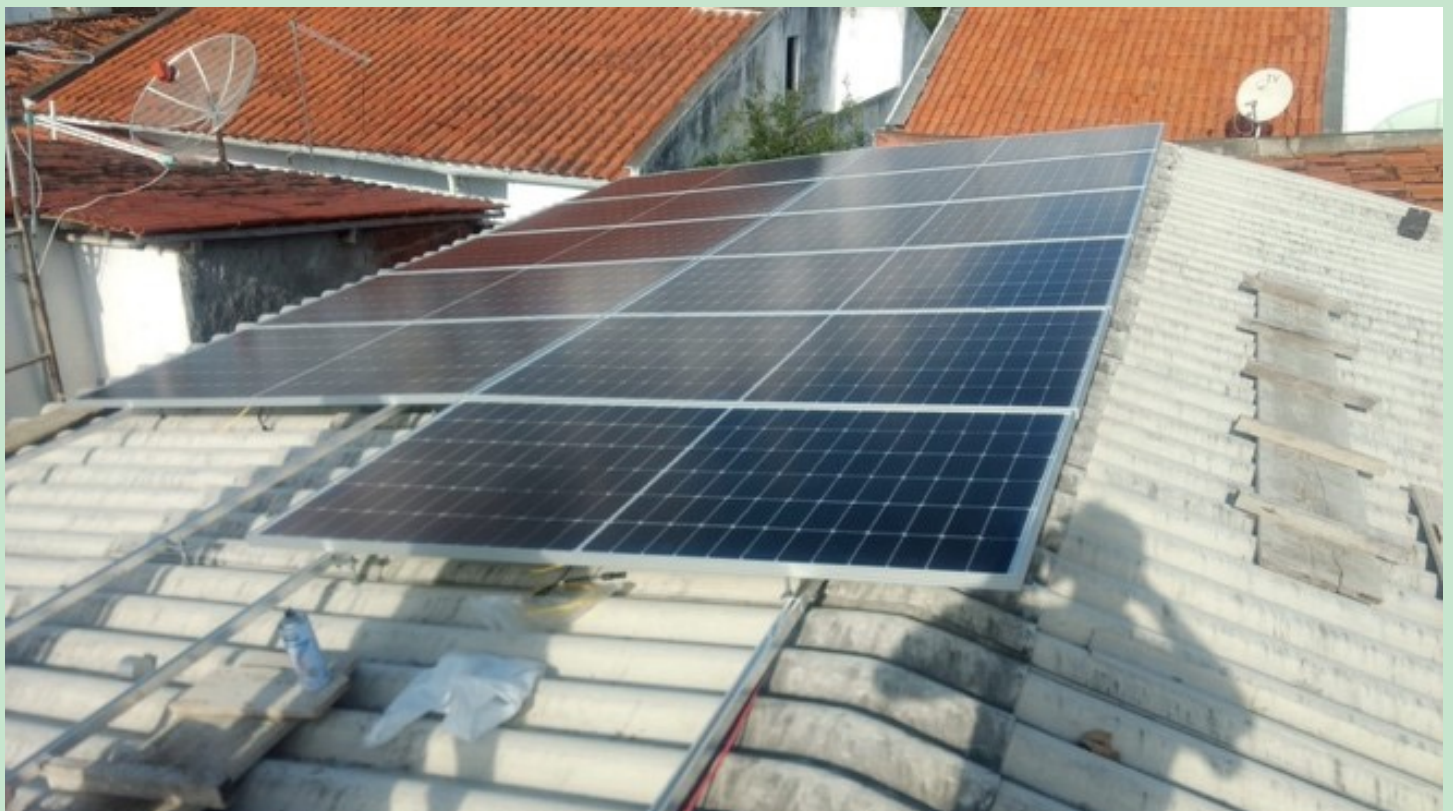
Solar panels installed in a roof/residential use (source: SOL Luções Energia Solar)
