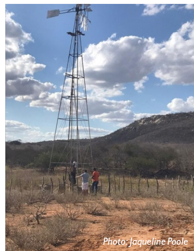
Fazenda Mares - São João do Cariri/Paraiba State rural area: an old windmill used to pump water
